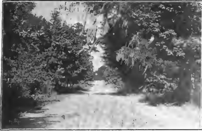
The new Waters road, ready for use
